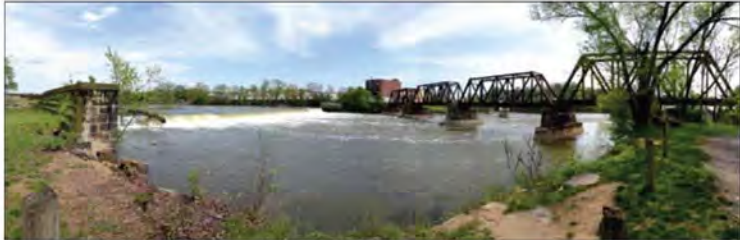
Panorama of the spillway and bridge on the Muskingum River in Zanesville.
