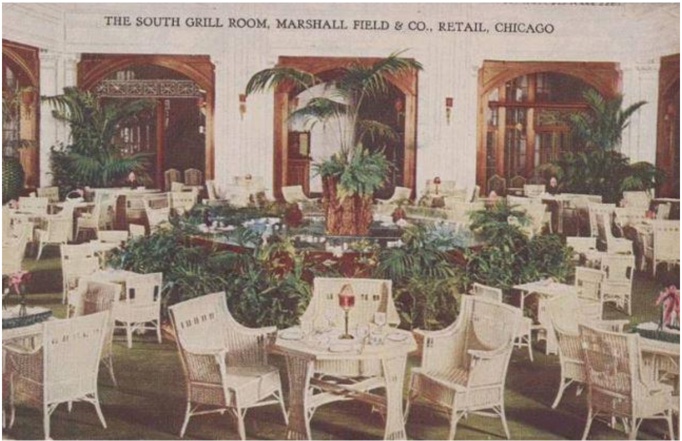
1907 view of the "South Grill Room"
